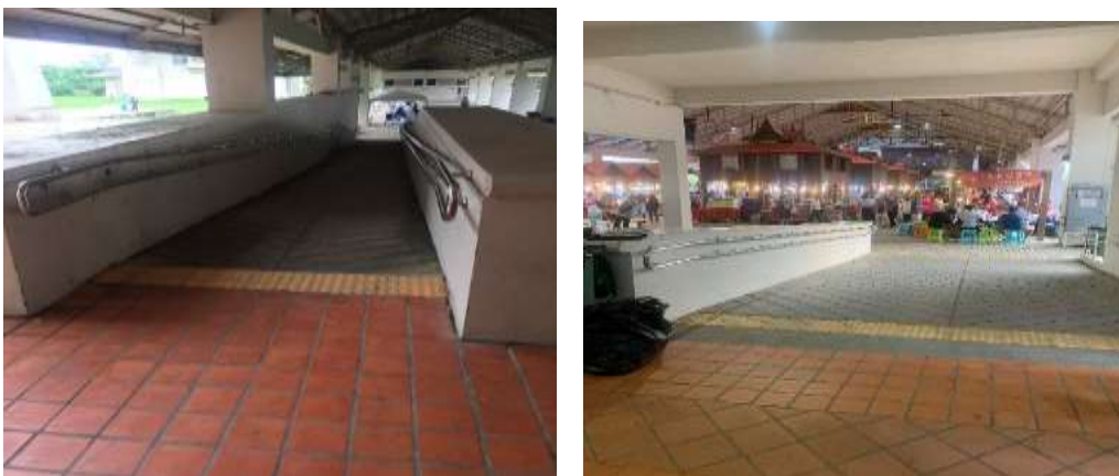
Figure 3. Internal pathway inside the building of Chiang Mai International Exhibition and Convention Center installed with ramps and handrails.
