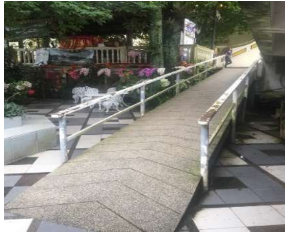
Figure 6. Ramp designed for the accessibility tourists at Phra That Doi Suthep temple.
