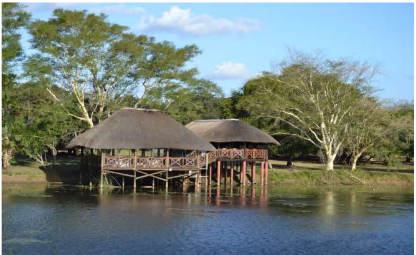
Figure 2: Conference room overlooking a dam at Bonamanzi Source: Author's own
