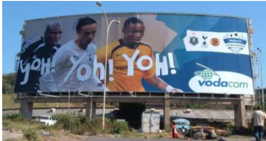
Figure 5: Gantry at Cape town for Vodacom
