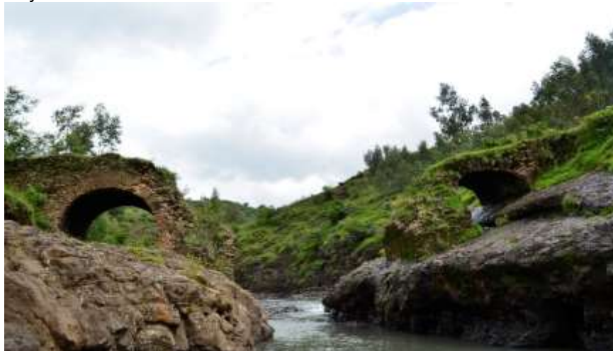
Bambilo Chigasa Bridge
